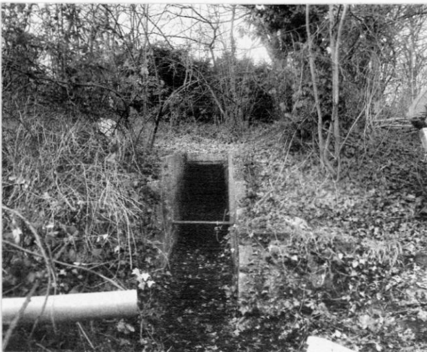
The current entrance to the mine.
